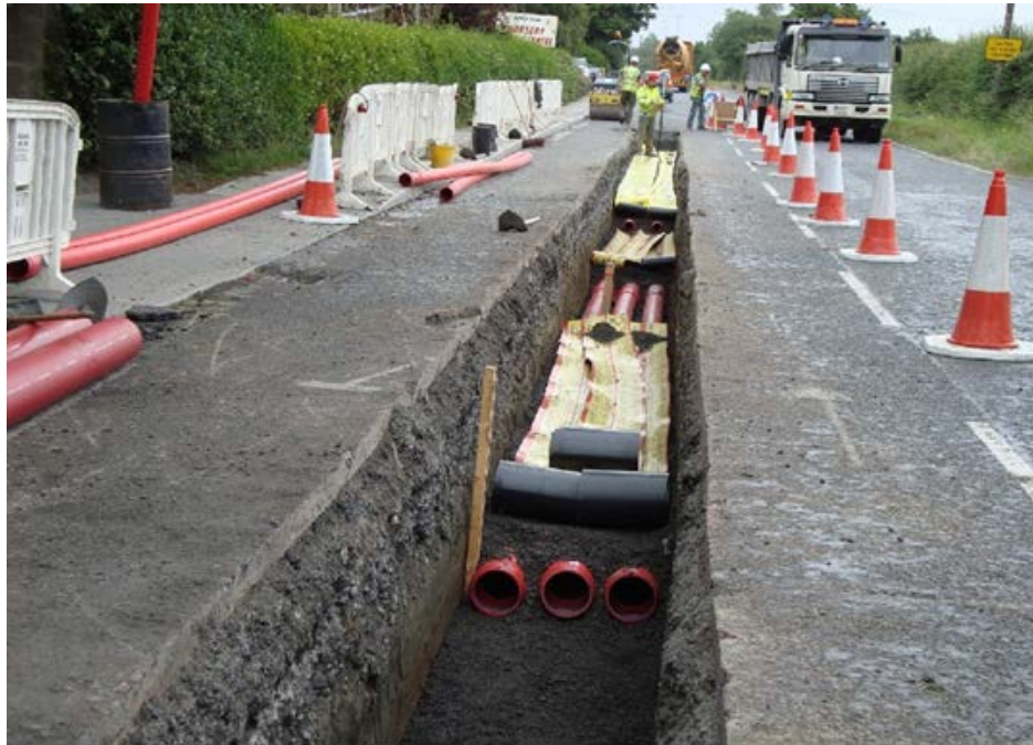
Plate 1 Example of UGC trench and ducting on public road.
