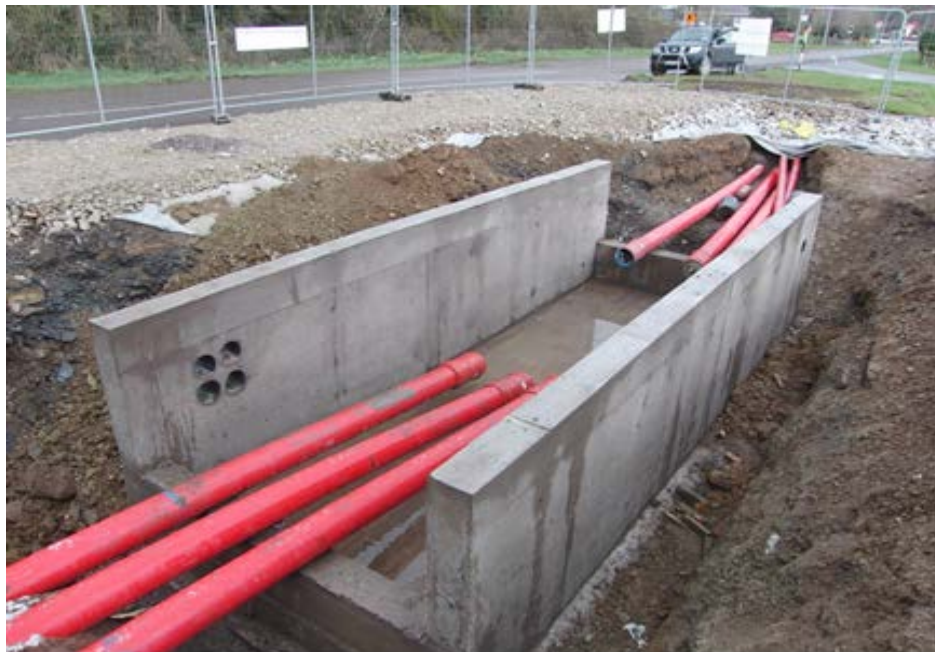
Plate 2 Example of typical UGC joint bay adjacent to public road.
